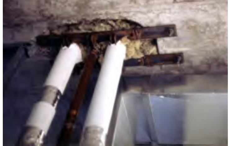
Source: Image by Wikimedia Commons user Achim Hering, accessed January 24, 2011, http://commons.wikimedia.org/wiki/File:Fancoil_unit_underside_of_firestop.jpg .
